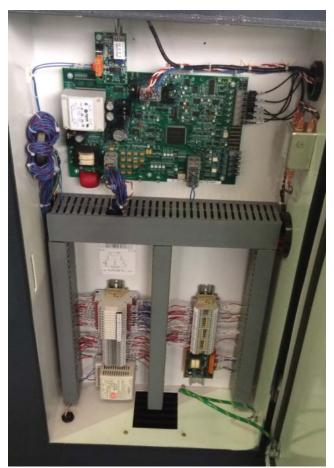
Figure 3- 5: Rectifier Logic Section
