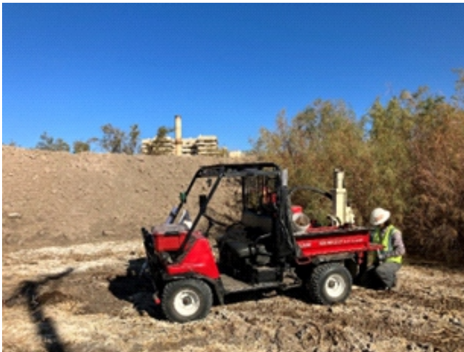
Photo 3: MW-3 and drilling B-3
